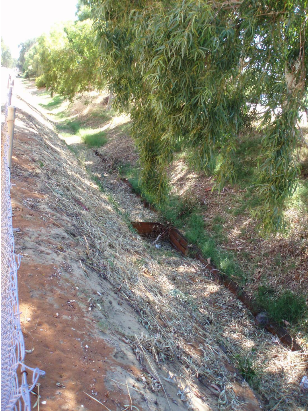
Figure 10: Section of Delwanee Drain showing decreased quantity of calcite pellets and exposed drain shoring (November 29, 2007).
