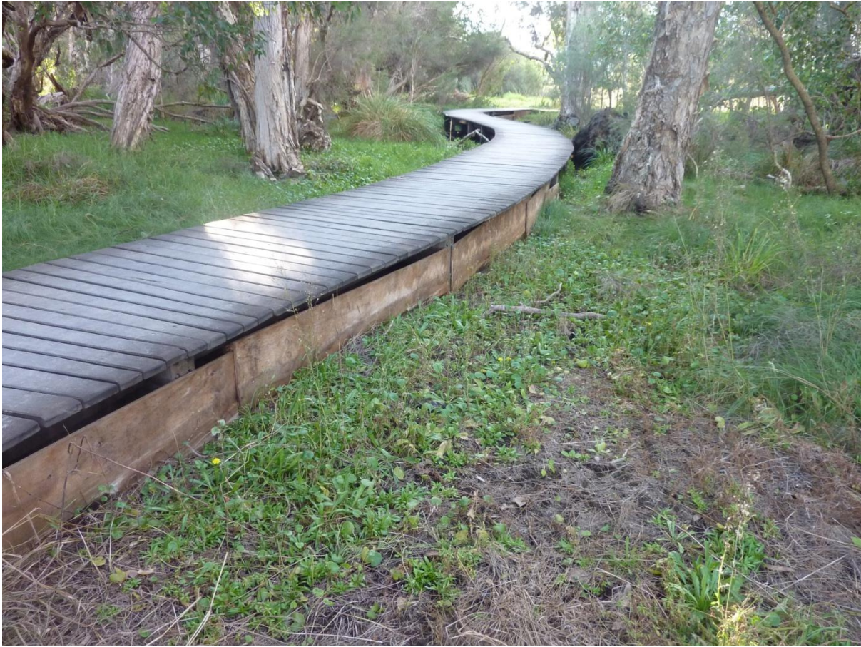
Figure 1. Beenyup Swamp input site, showing the boarding used to target and control flows for more accurate determination of flow volumes
